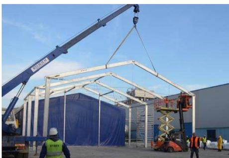
As the framework is being erected the steelwork that forms the join between frames will be placed. All of the work at height will be conducted from a suitable platform, either a MEWP or scaffold in accordance with WAHR.
